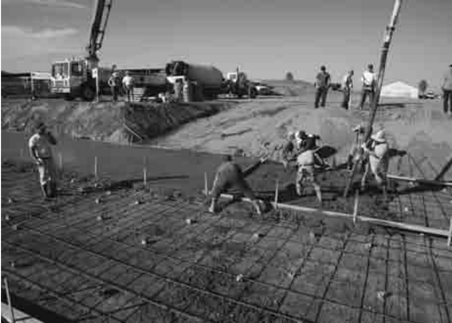
Plate 11.1 Dairy barn expansion
